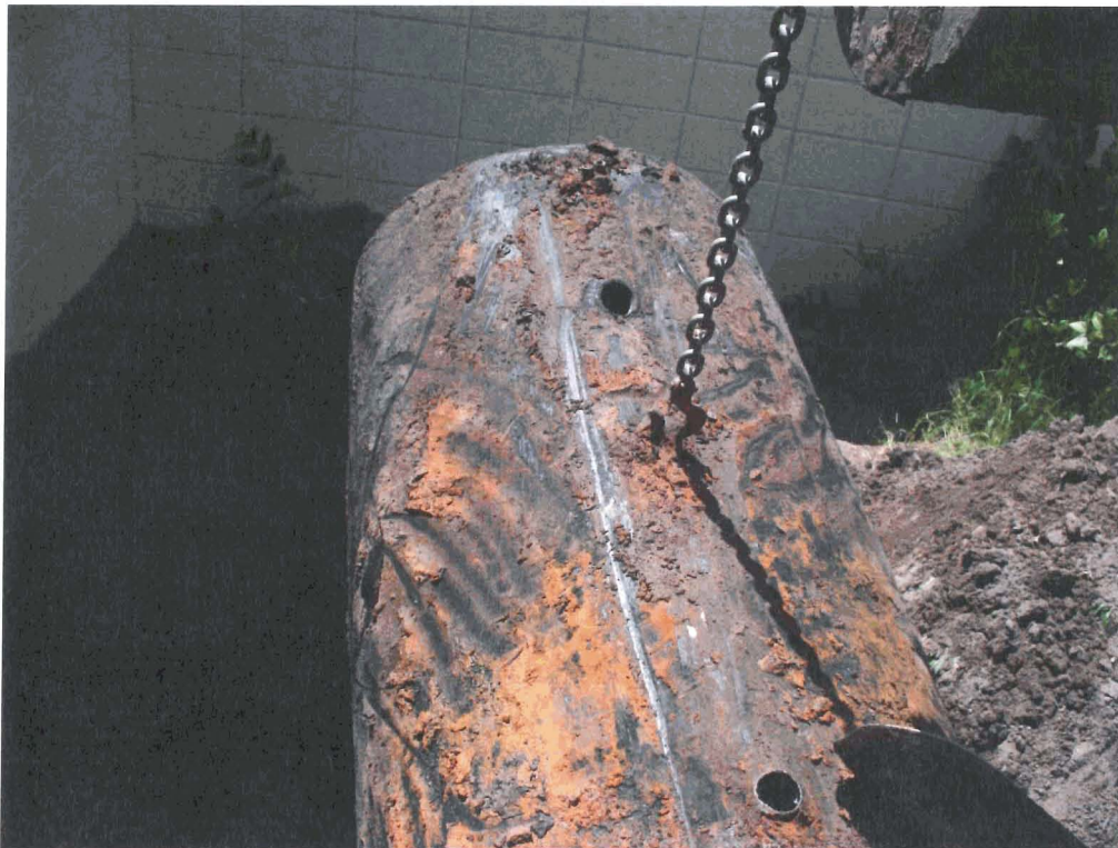
Picture 2: UST 644Dahlia-1 being removed from the excavation.
